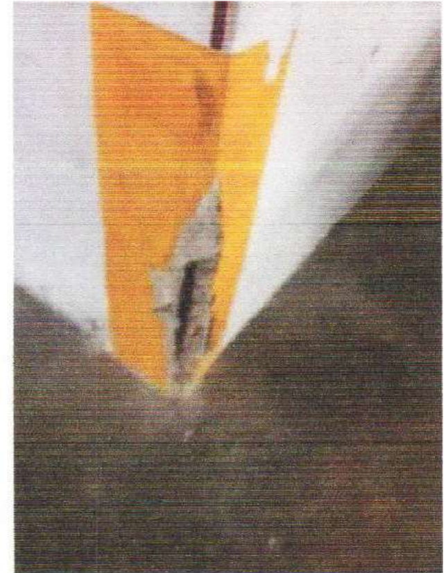
Figure J1: Typical cracking and spalling at parking garage columns
