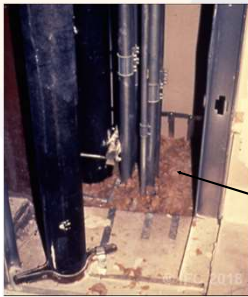
Fire blocking or safing with wool
